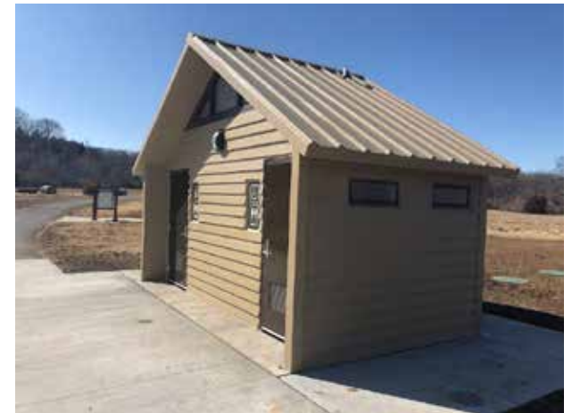
Structured restrooms are preferred, but Porta-a-potty restrooms can also fill a need at a trailhead.
