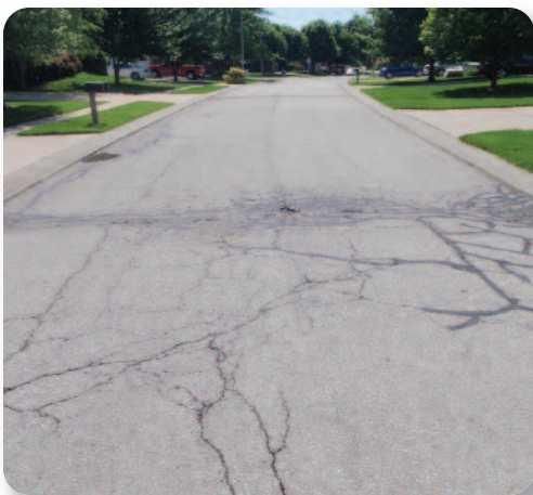
W. 158th Street – Before 2016 Mill and Overlay
