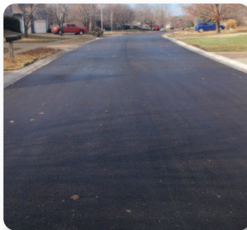
W. 158th Street – After 2016 Mill and Overlay
