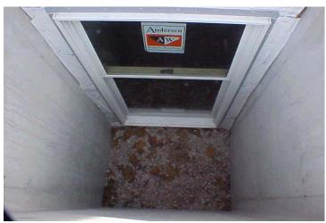
18 inches on center vertically for the full height of the window well If a cover is provided over the well it shall be openable from the egress side and provide the same clear areas as require for the window.
