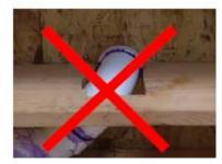
Bored holes in engineered wood trusses and I-joists
