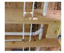
**Top of Wall Support / Isolation** – The tops of walls should be attached to the supporting framing above to provide lateral support. Some cities require that nonbearing walls provide an isolation joint at the top of the wall (hold the wall below the bottom of the floor
