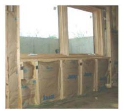
**Wood framed walls** (including the joist cavity at the rim joist) shall be insulated to provide a minimum R-13 insulation.
