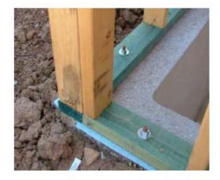
**Wall Sole (Bottom) Plates** – The wood sole plates which are not separated from the slab by an approved moisture barrier (such as a polyethylene plastic 6 mils or more in thickness) are required to be pressure treated or naturally decay resistant wood. Studs or other framing members in direct contact with a concrete foundation wall also are required to be pressure treated or naturally decay resistant wood.
