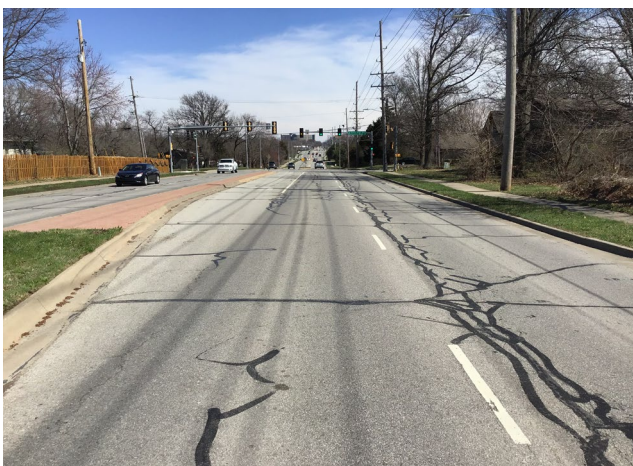
Rubberized Asphalt Crack Seal
