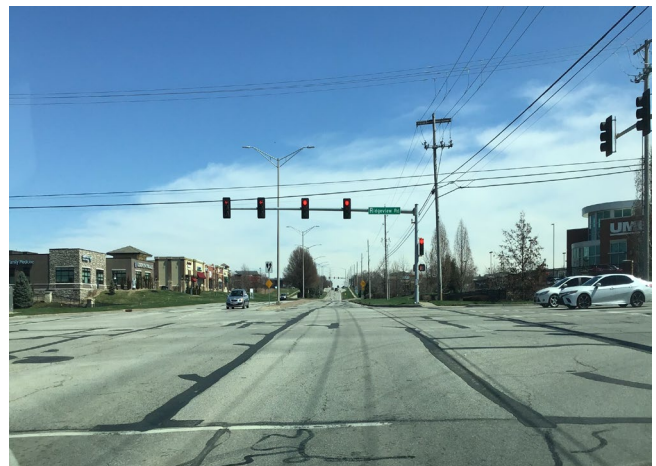
Wide Asphalt Crack Seal
