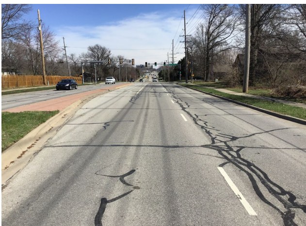
Rubberized Asphalt Crack Seal
