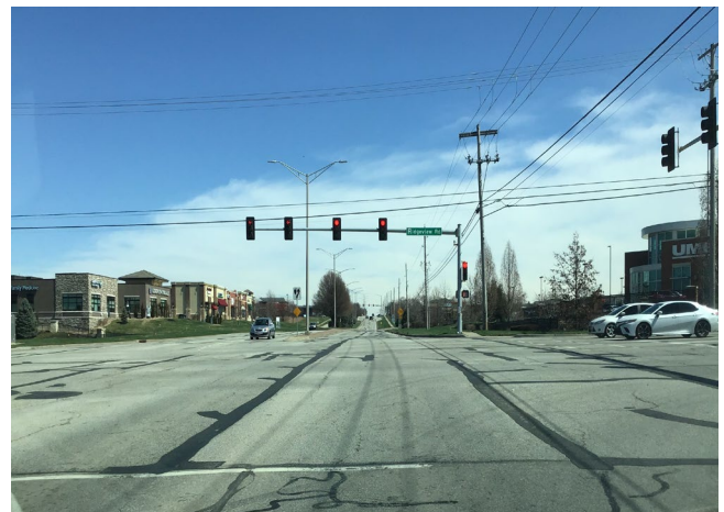
Wide Asphalt Crack Seal
