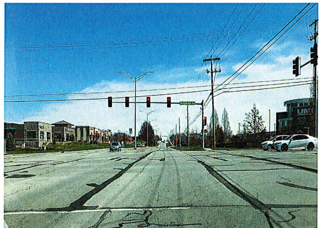
Wide Asphalt Crack Seal
