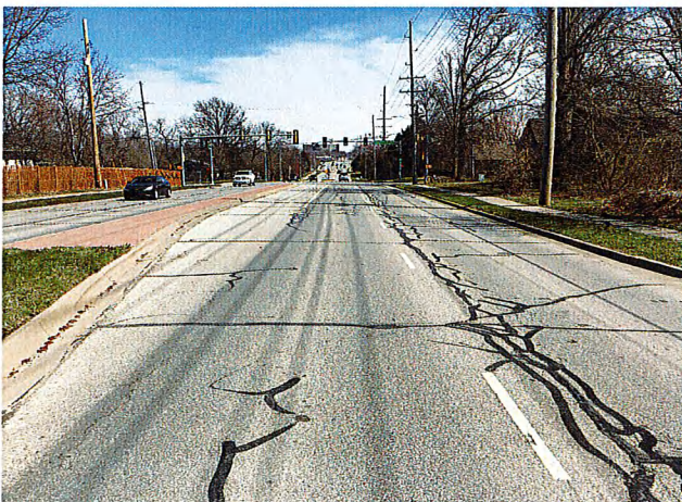
Rubberized Asphalt Crack Seal
