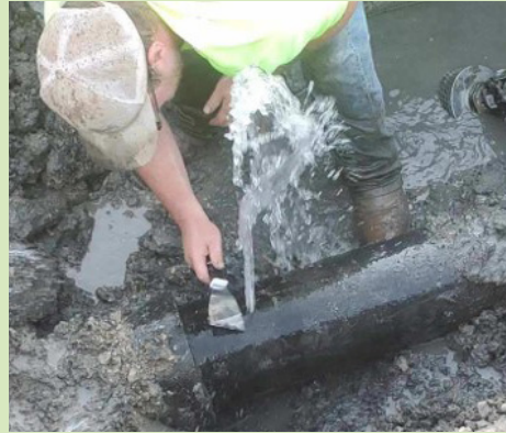
Cody Springston, scrapes the water main before installing a repair band.
