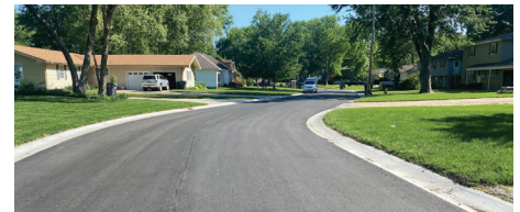
After street maintenance
