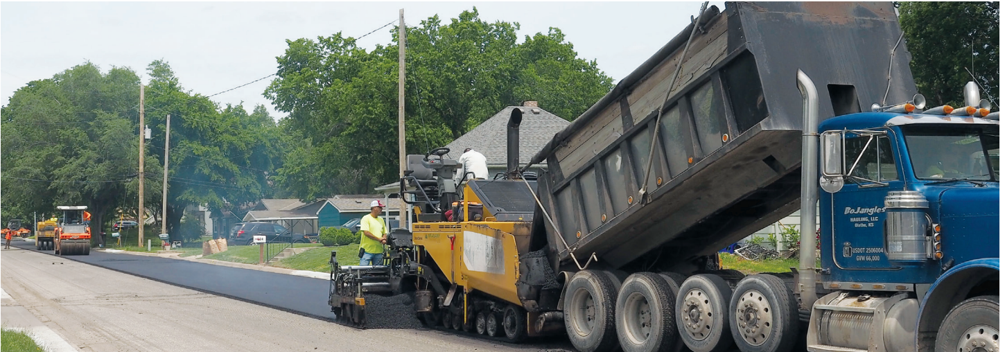
Crews placed new pavement on Iowa Street in May 2022.
