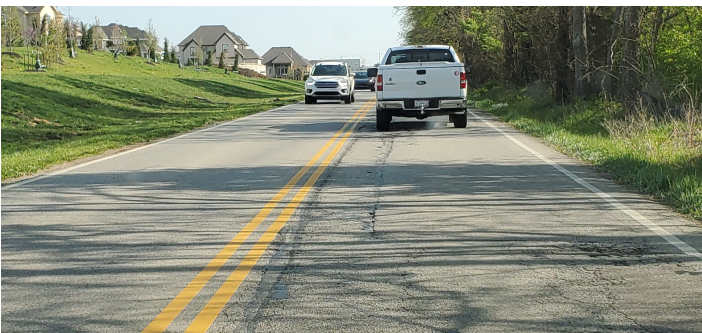
Existing Pflumm Road
