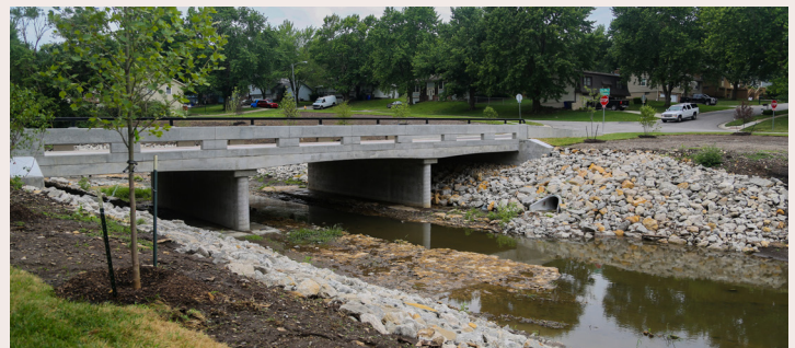
The improved Northview Street bridge over Mill Creek, near Parkway Drive and Harold Street, combined with other channel improvements has reduced the risk of flooding to the area.
