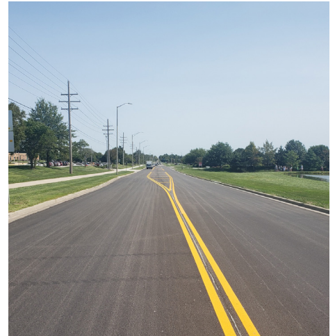
159th Street AFTER new pavement in 2021
