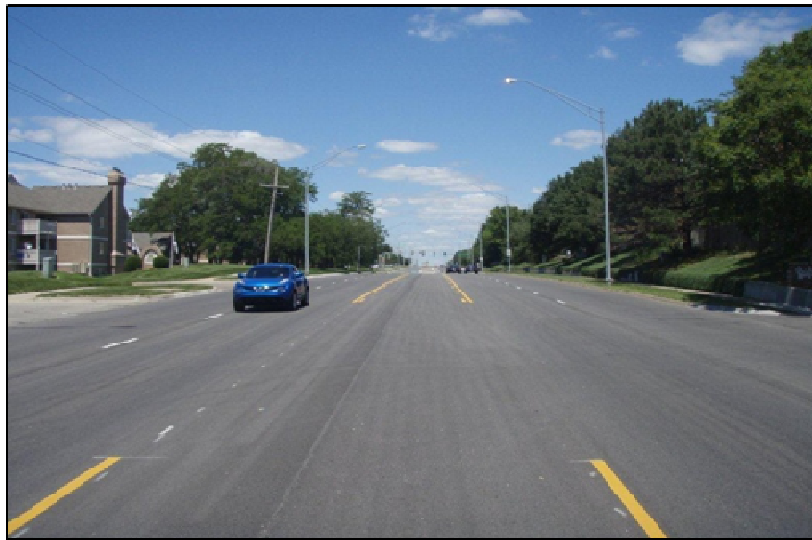
Completed Street Preservation project
