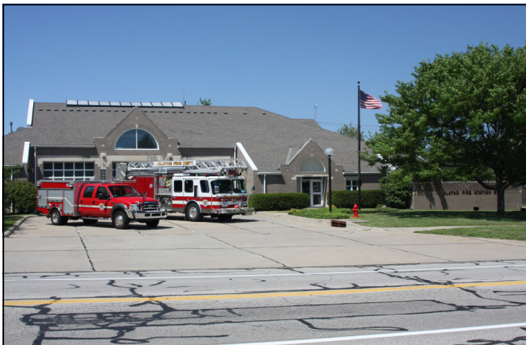
Fire Station Maintained by Building Maintenance
