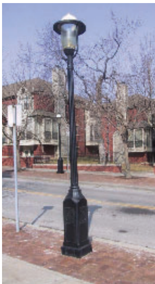
Combined pedestrian and street lighting
