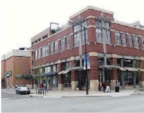
Parking structure with retail on ground floor, quality materials, and detail
