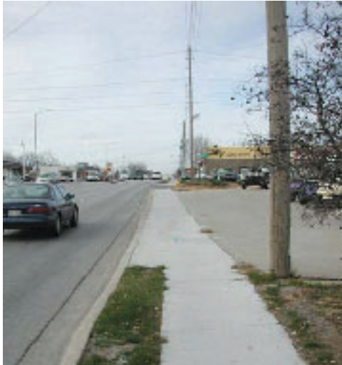
Large existing curb cut
