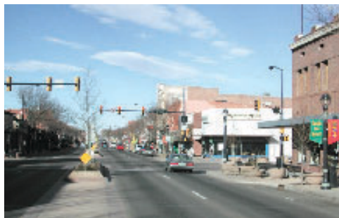
Example of Santa Fe Corridor character with median, curb extensions, street trees, pedestrian lighting, on-street parking, and street furniture
