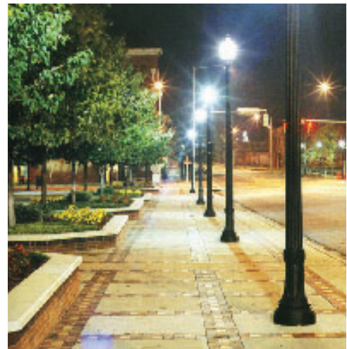
Pedestrian lighting that provides street lighting
