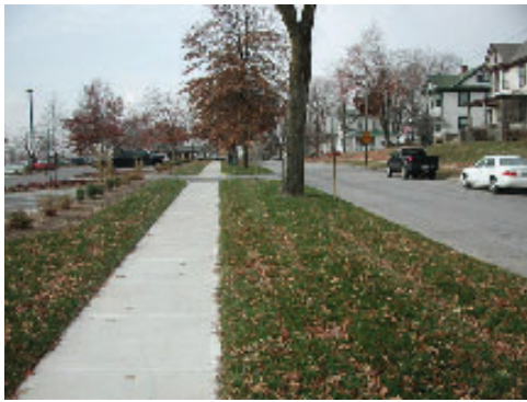
Poplar Street transition area
