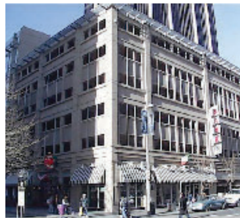
Active uses at street level of parking structure and high quality facade
