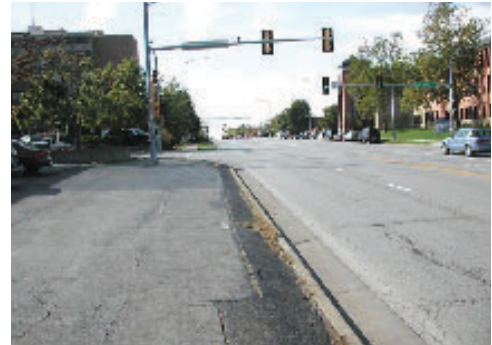
Existing Santa Fe Street at Chestnut Street
