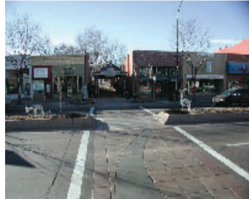
Example of midblock crossing treatment with a pedestrian refuge in the center
