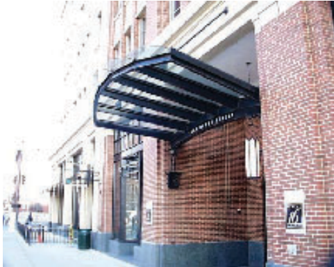
Emphasis on building entry
