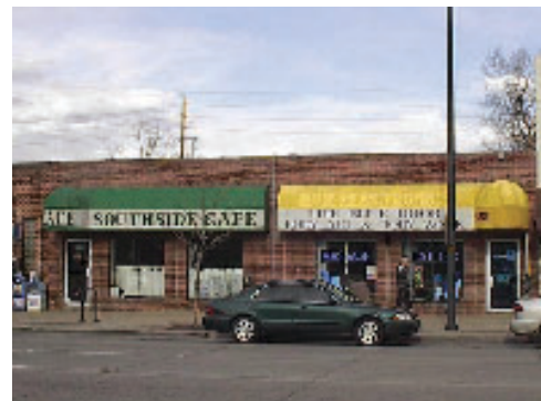
Undesirable barrel awning
