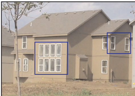
Rear wall windows and side wall windows
