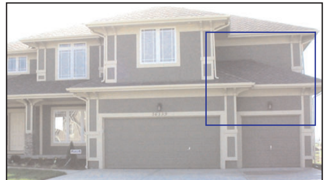
The garage roof(s) appears to be integrated into the main portion of the structure's roof
