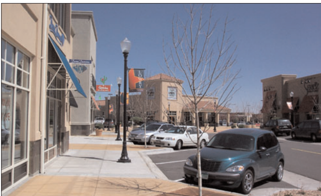
Mixed-use areas provide the ability to integrate retail, professional office and attached residential within a single development.
