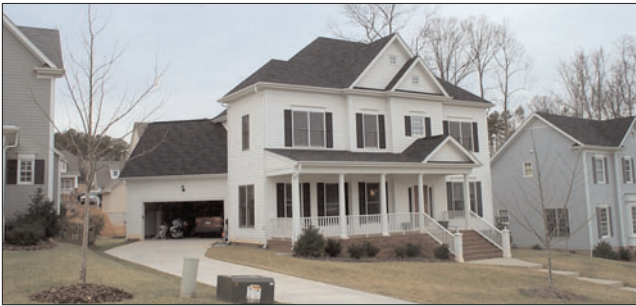
Garages should be set back from the front elevation. When possible, alleys should be utilized with rear loaded garages.
