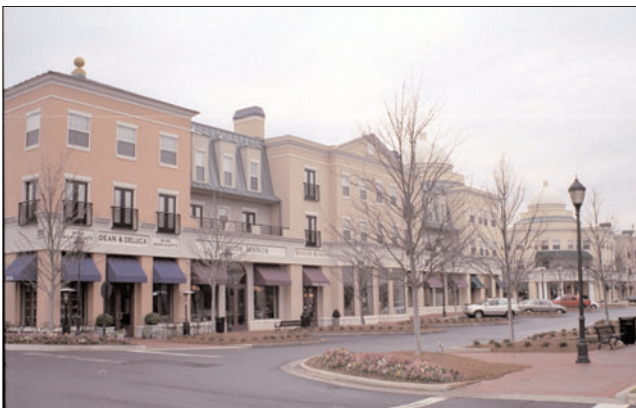
Building heights should be up at least two stories with the front façade addressing the street.
