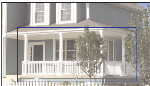
Large porch on two sides of structure
