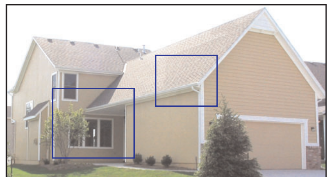
Painted trim on all sides of the structure and multiple exterior wall offsets and projections
